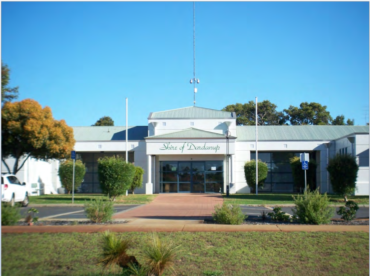
Dardanup Shire Council – Eaton Administration Centre
